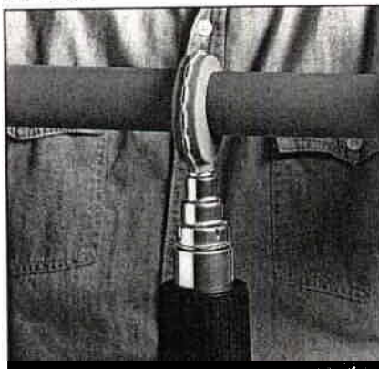
Welding with heat reflector
